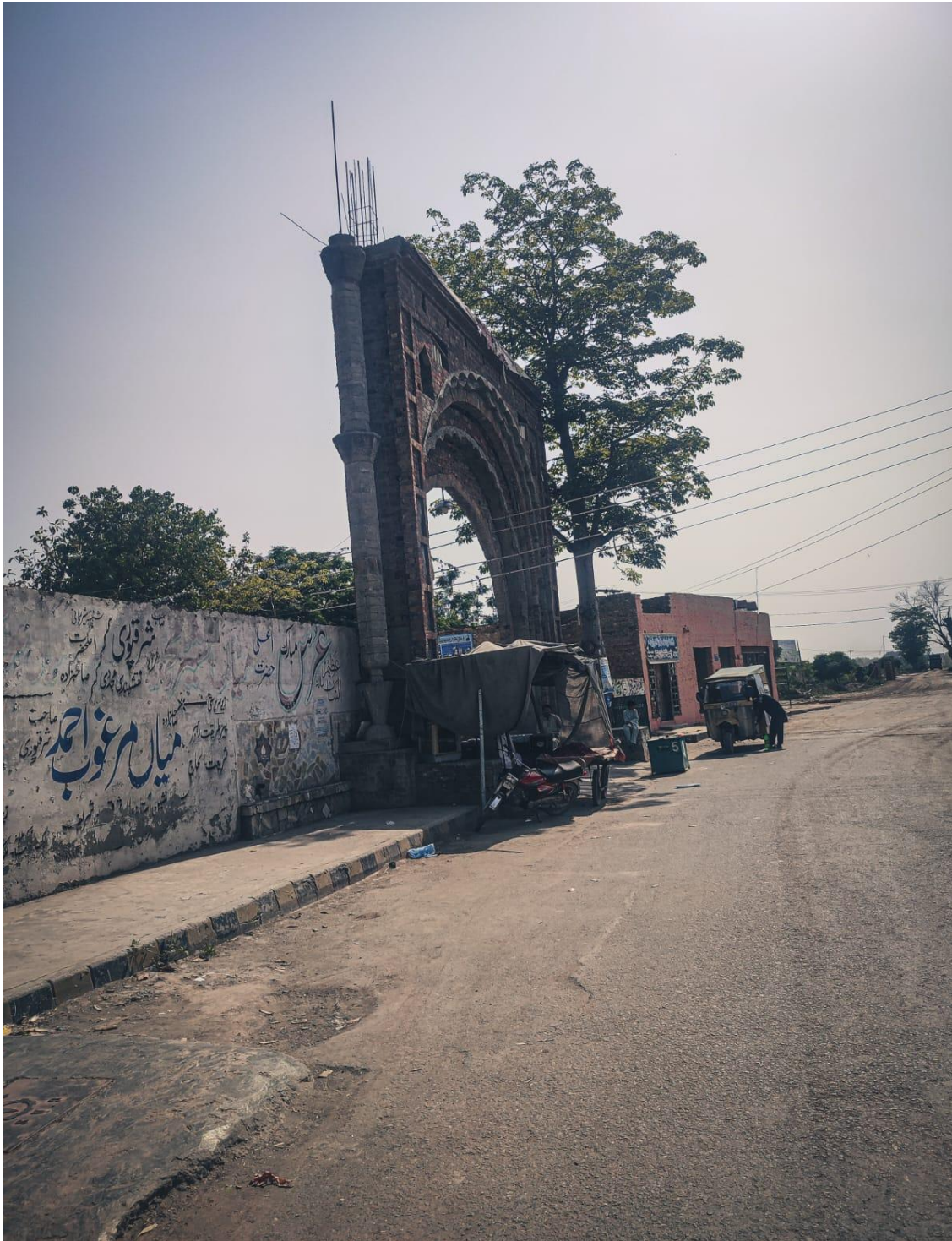
Figure 1: This is the road that leads to the shrine. The incomplete structure of bricks and concrete is the first entrance of the shrine. There are some stalls on both sides of the entrances.
