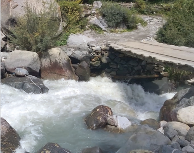
Image 7.2 Gilgit Baltistan hand-made bridges of wood planks
